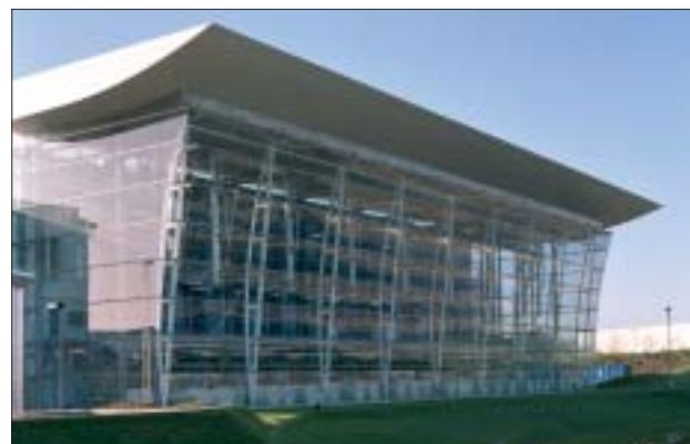
Independent Newspapers: Dirivent Air Conditioning System.
