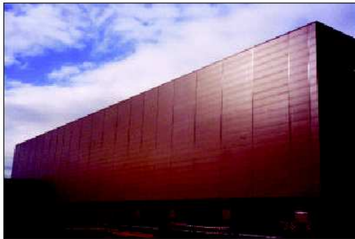
Wyeth Medica's high-bay warehouse for pharmaceuticals in Newbridge, Ireland.
